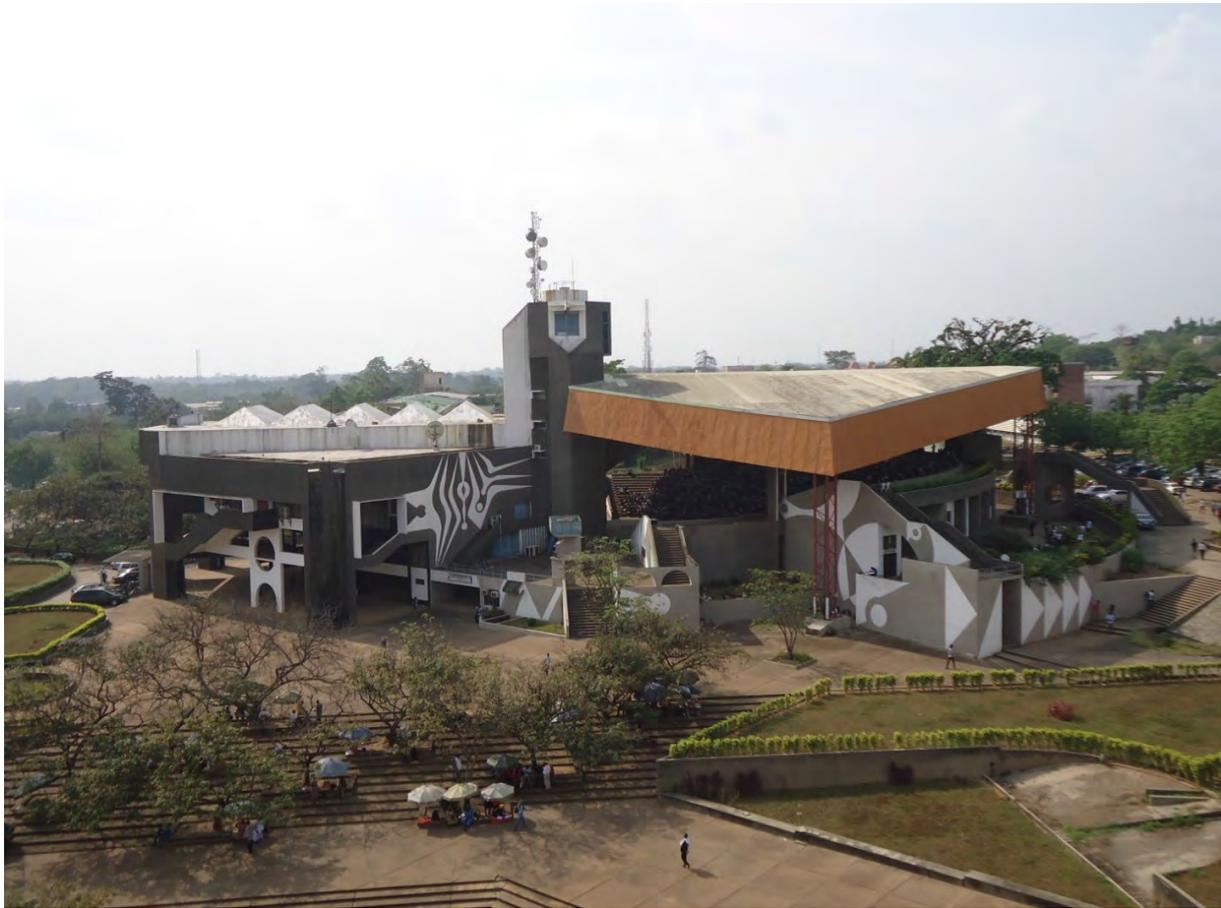
Figure 3. Oduduwa Hall, Obafemi Awolowo University, the Greek agora formed amphitheater, the original open air amphitheater is now covered with an aluminum roof (Source: Authors).
