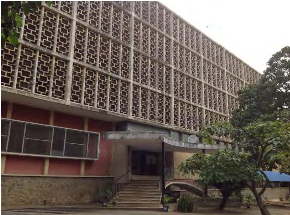
Figure 6: Kenneth Dike Library, University of Ibadan showing the reinforced concrete screen wall patterns juxtaposed with the international style influences (Source: Authors).
